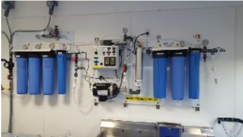
Miniaturized wastewater treatment systems for removal of small quantity hazardous materials, precious metals reclaim and other small scale operations that do not require large, expensive water treatment systems, but need automated, reliable equipment to keep operations running smoothly.
