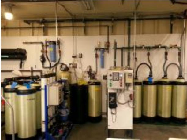
Service tanks for high purity, spotless rinse and other applications, deionized water systems and central purified water and sterile water systems for applications in manufacturing, cosmetics, cleaning, food and beverage and other critical process where consistency and non-reactive water are important.
